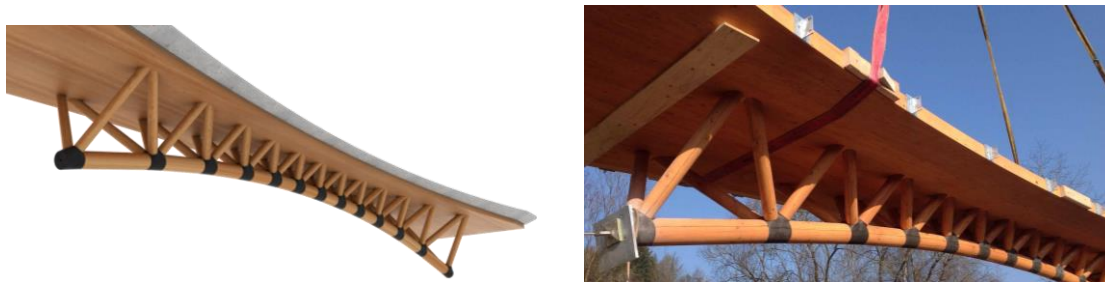
Figure 3: Composite timber truss bridge with grouted joints
