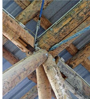
Figure 1: Conventional round-to-round timber joint
