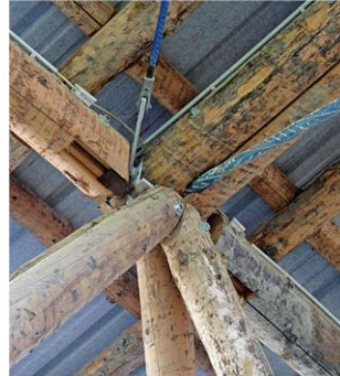
Figure 1: Conventional round-to-round timber joint
