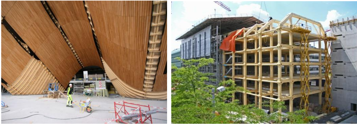
Figure 6: The wooden Wave as a free Form, Kristiansand, Norway, Tamedia office building: 5-storey building in Zürich, Switzerland [6]
