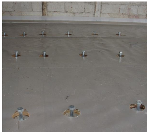
Figure 11: Strengthening of existing timber beam ceilings with TCC; left: typical building with timber beam ceilings, right: arranged ceiling before casting
